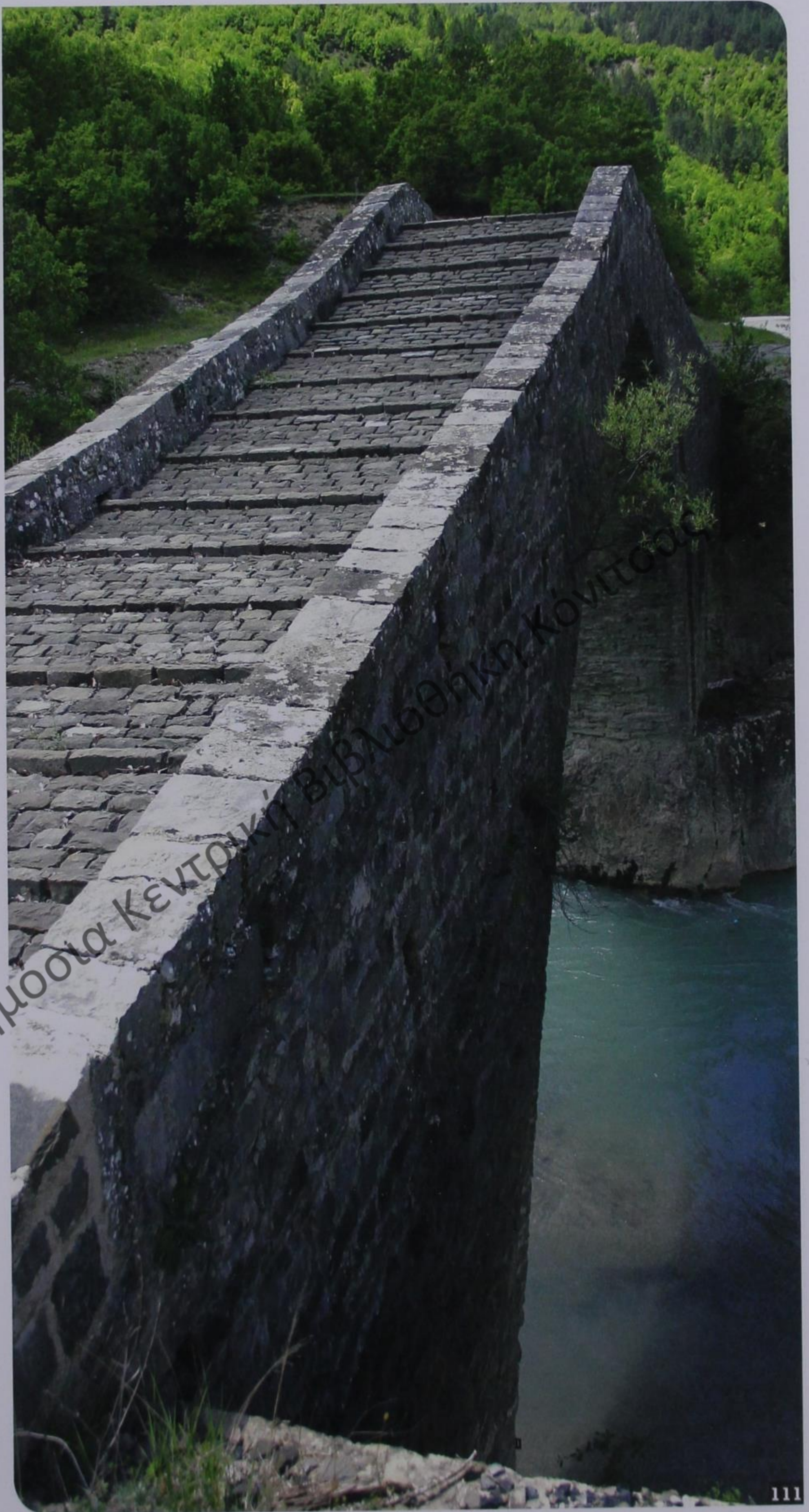
11: The Kantsiko bridge in Drosopigi is of outstanding importance, since it is the only bridge nowadays that still connects the mountain villages from both sides of Sarantaporos
