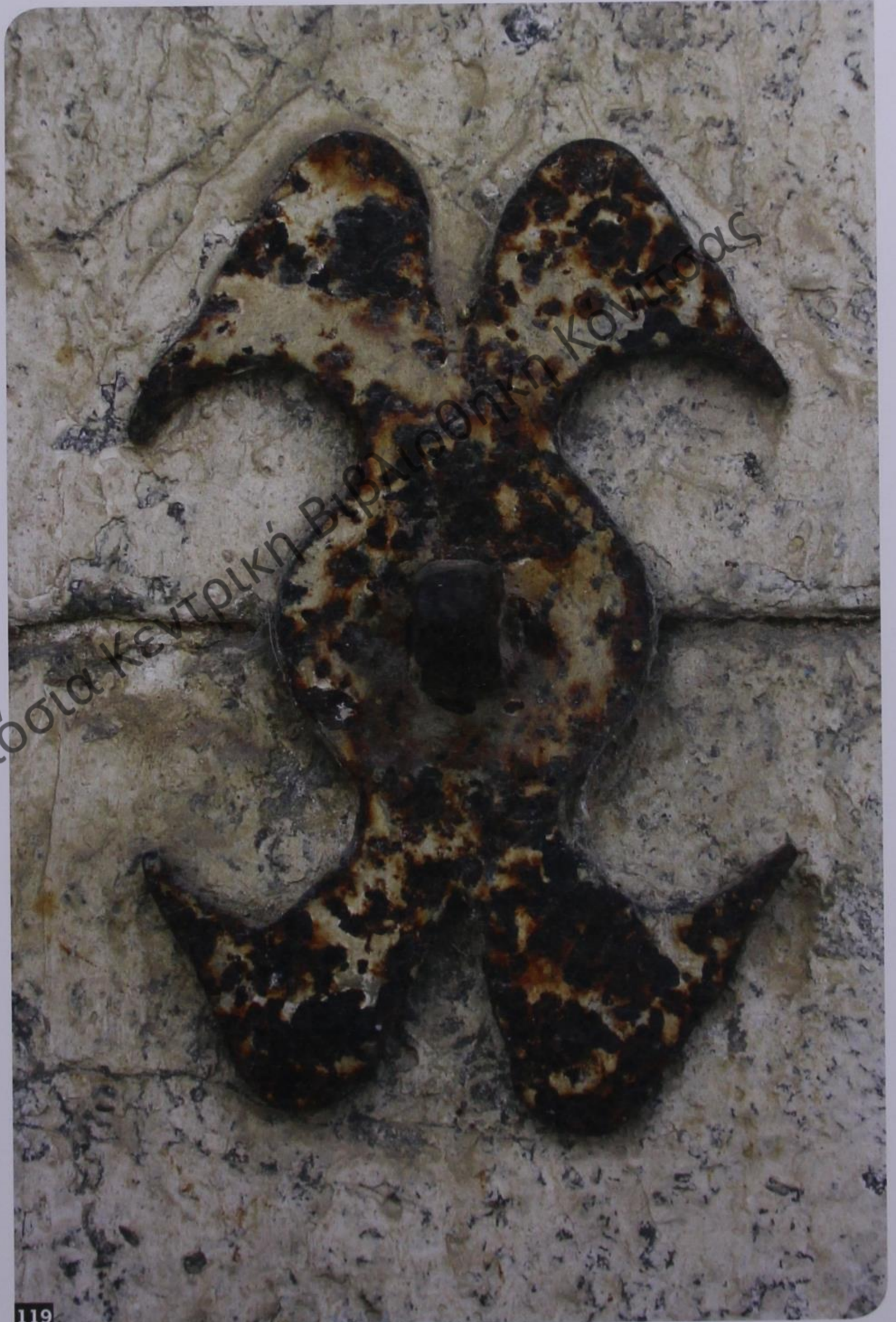
119: Exohi. Even the smallest structural details have a great aesthetic value
