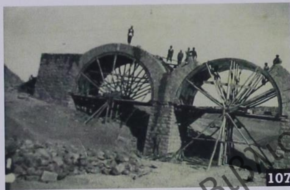
108: Detail of the construction of the bridge for the Railway in Teheran, 1936. Detail (Petronotis & Papageorgiou 2008:493)
