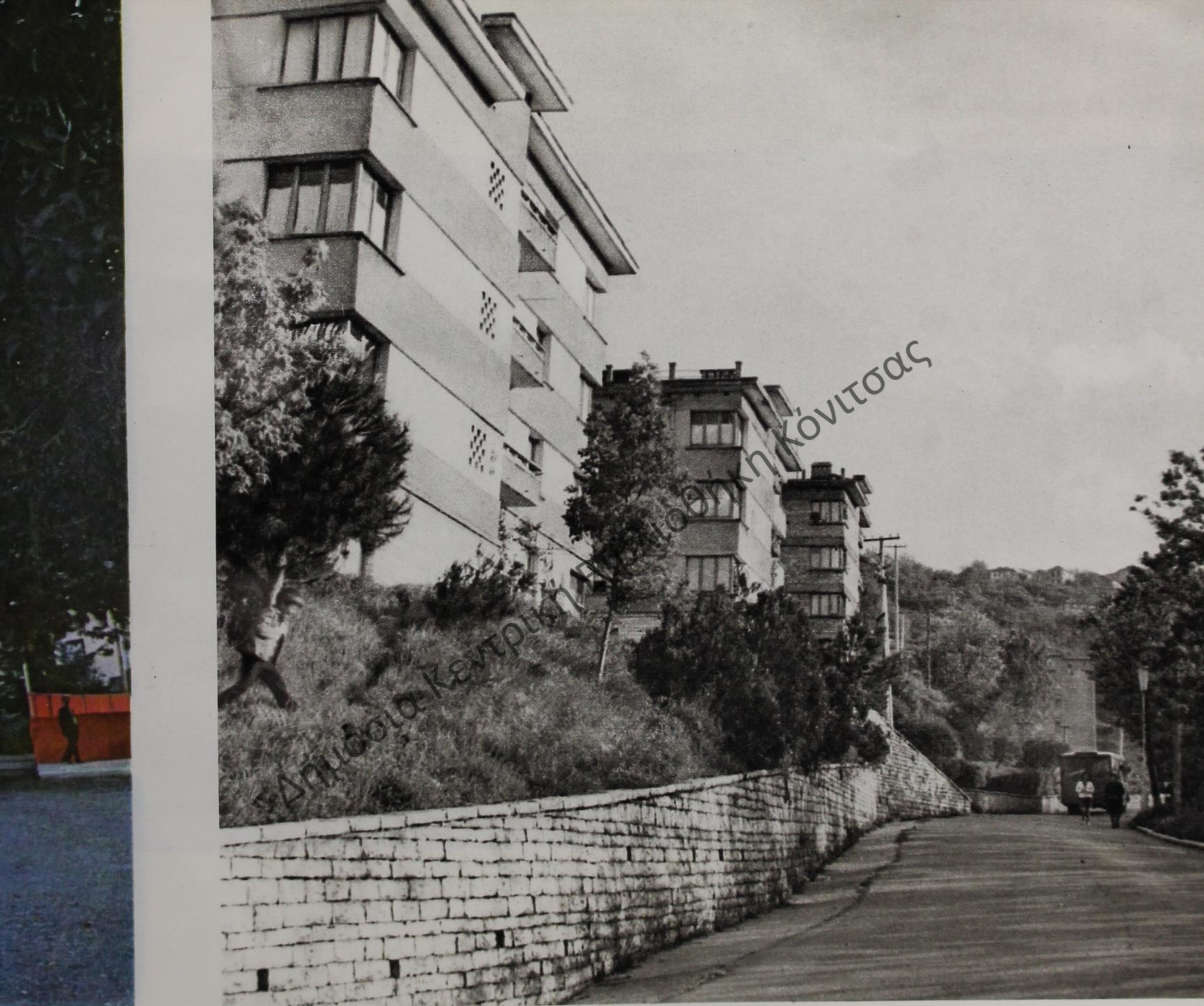
New constructions in the free zone.
