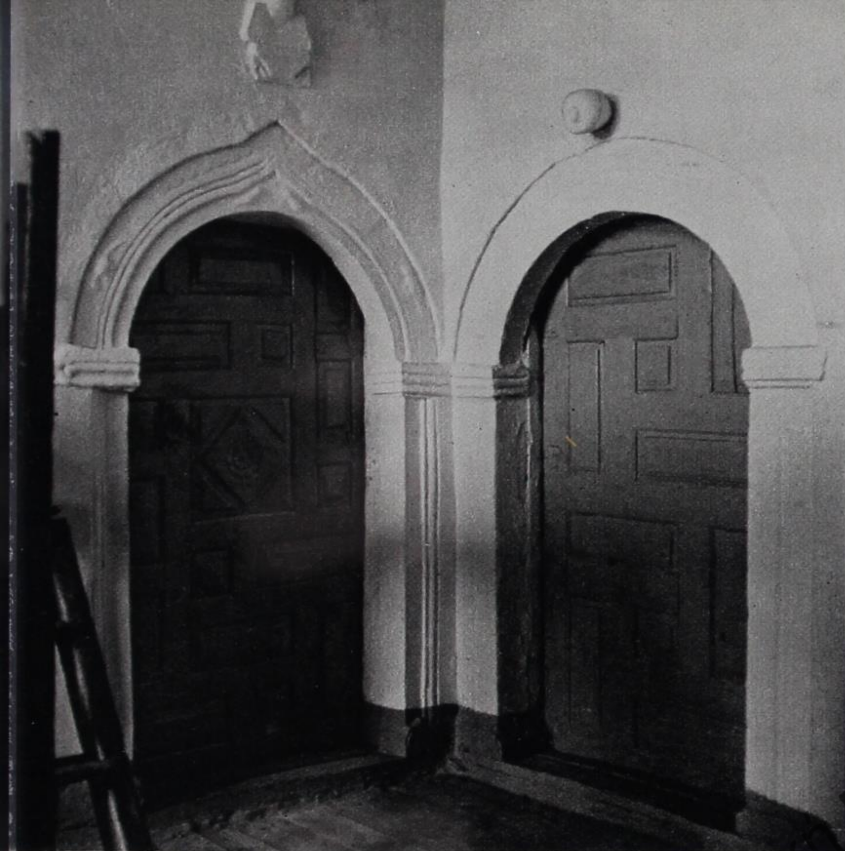
The Manalat quarter. The inner doors leading to the veranda.
