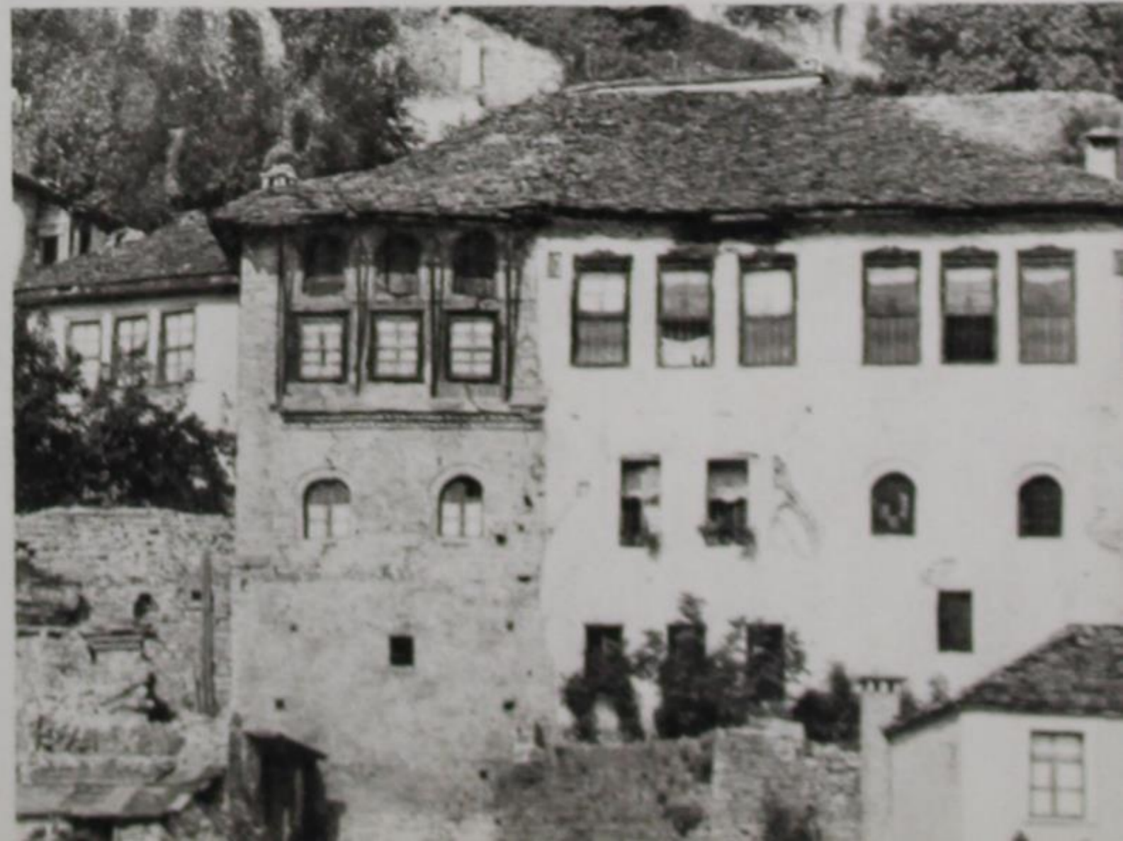
A dwelling-house in the Tekke quarter (before its restoration).
