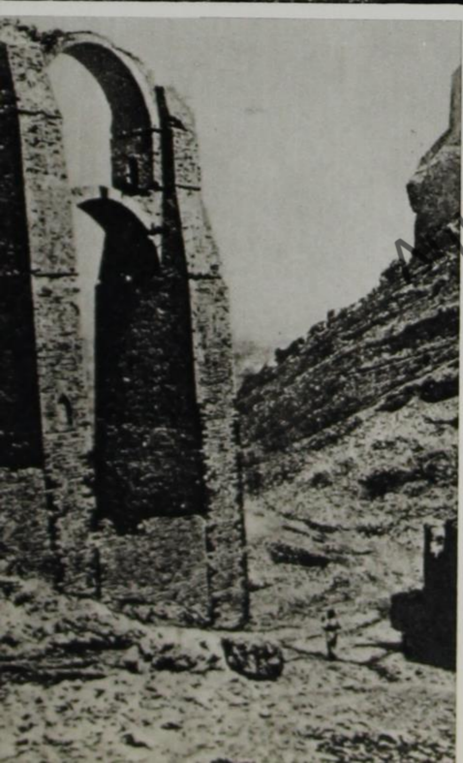
A partial view of «The Great Bridges» destroyed in 1932.
