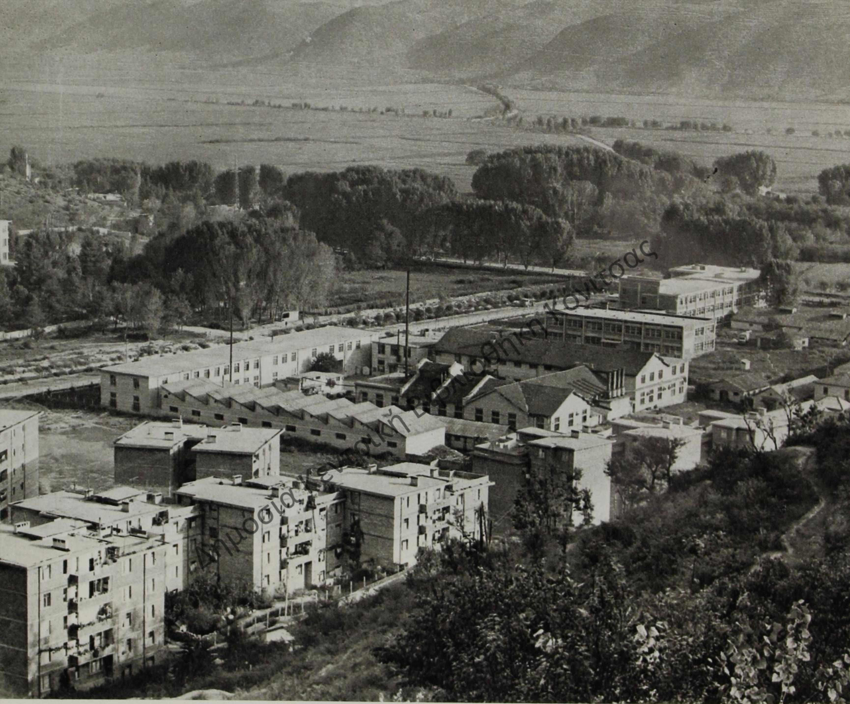
New constructions in the free zone of the museum city.
