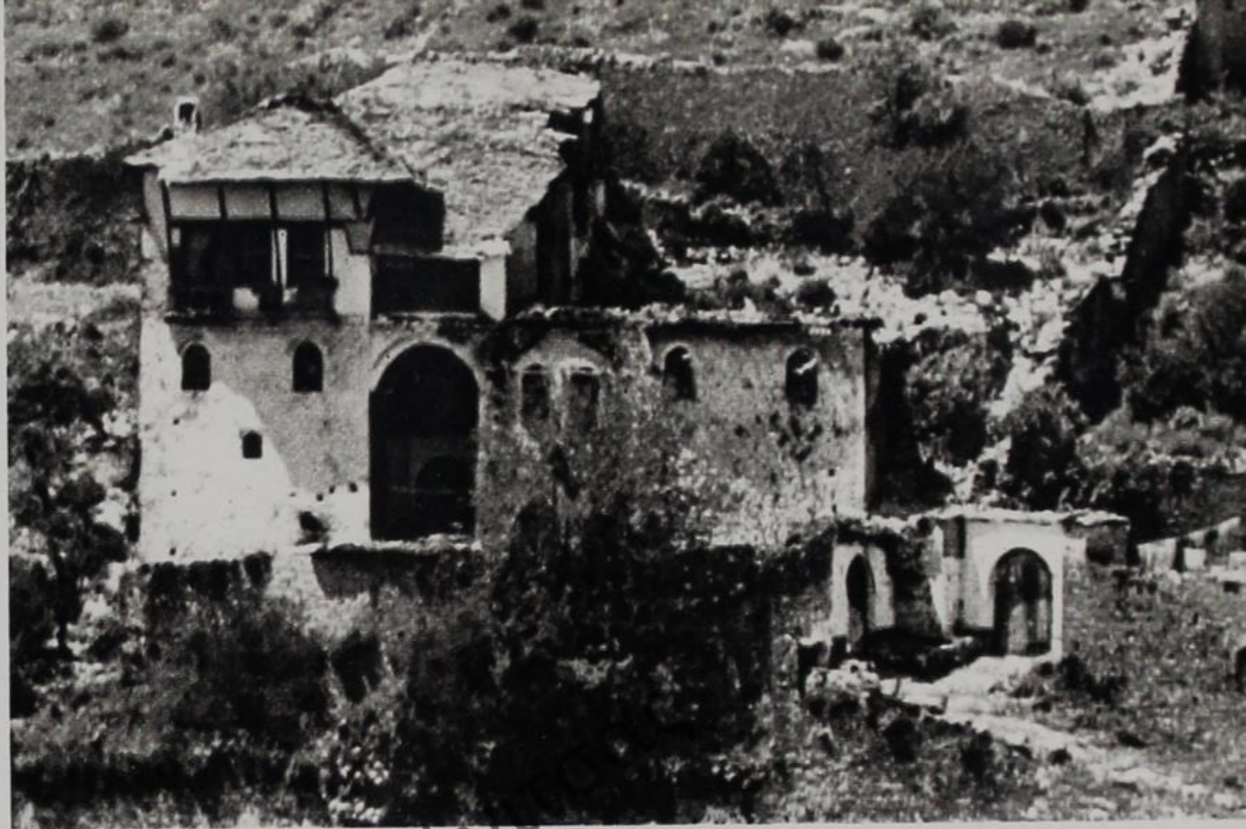
A dwelling-house in the Tekke quarter (before its restoration).
