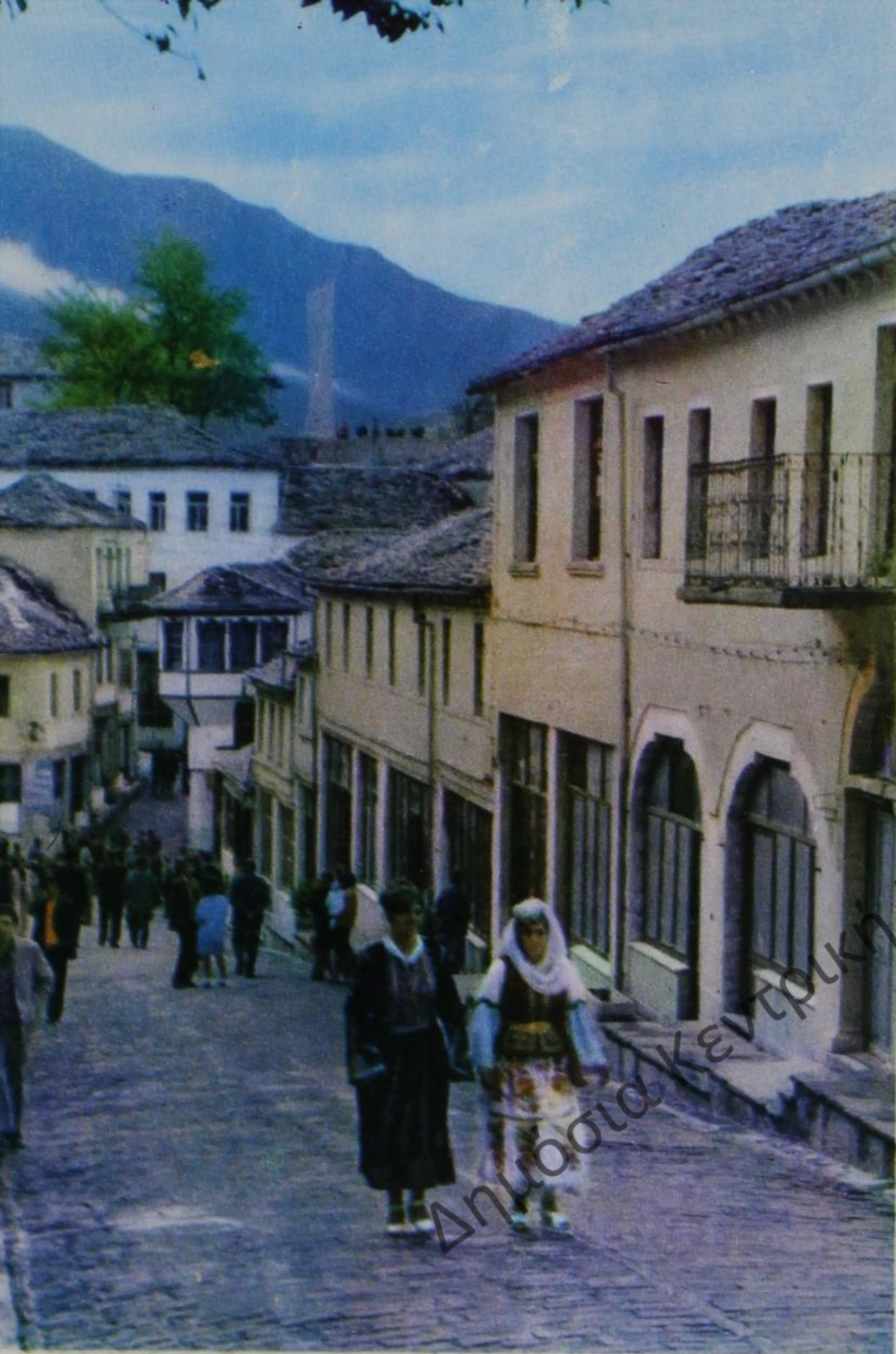
«The Bazaar Pass» (after its restoration).
