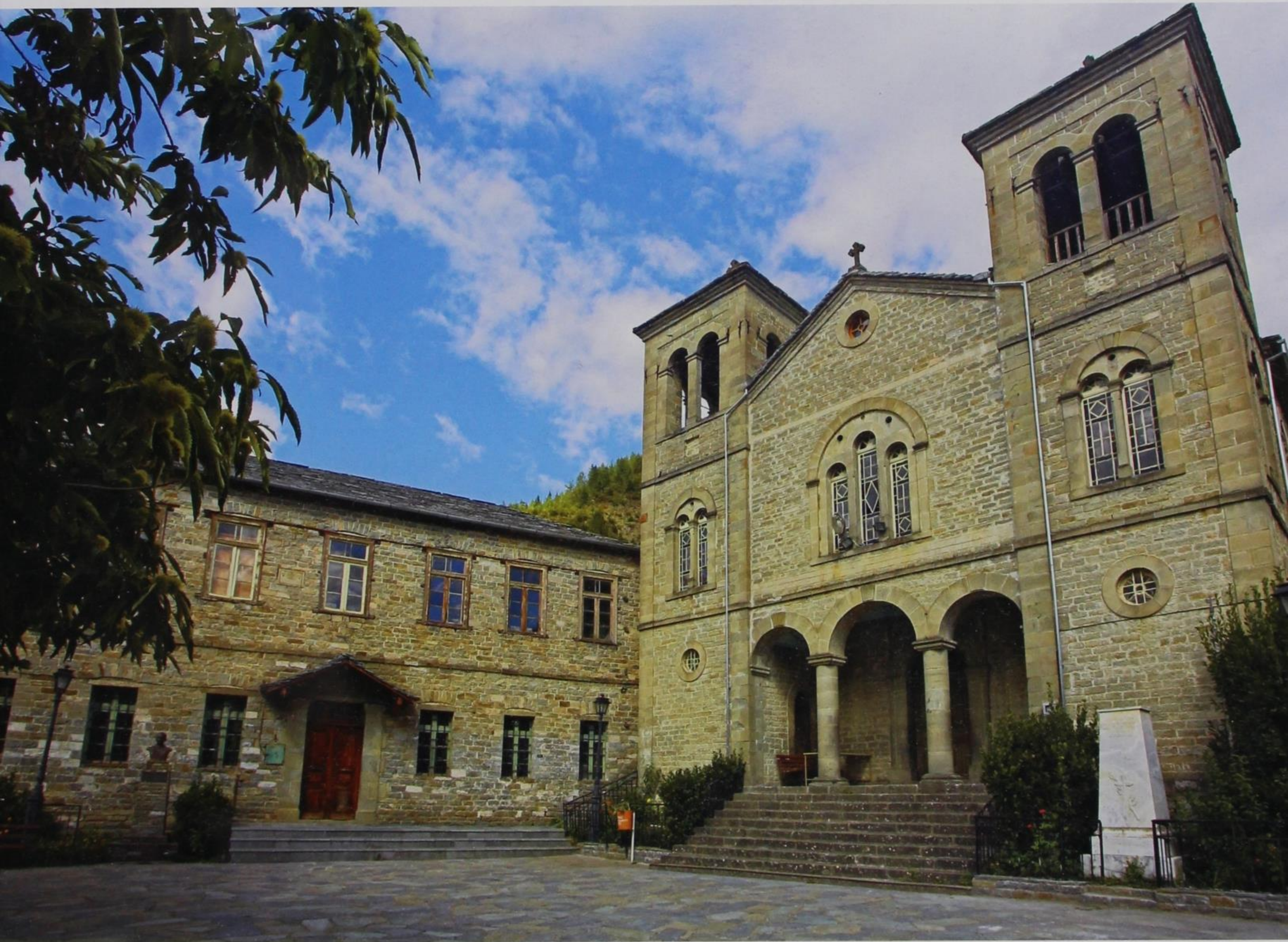
The craftsmen of Kastaniani applied their architectural and technical skills in the construction of public and private buildings in their village. On the left, manor houses of the village and on the right the Cathedral of St. Nicholas and the Elementary School.
