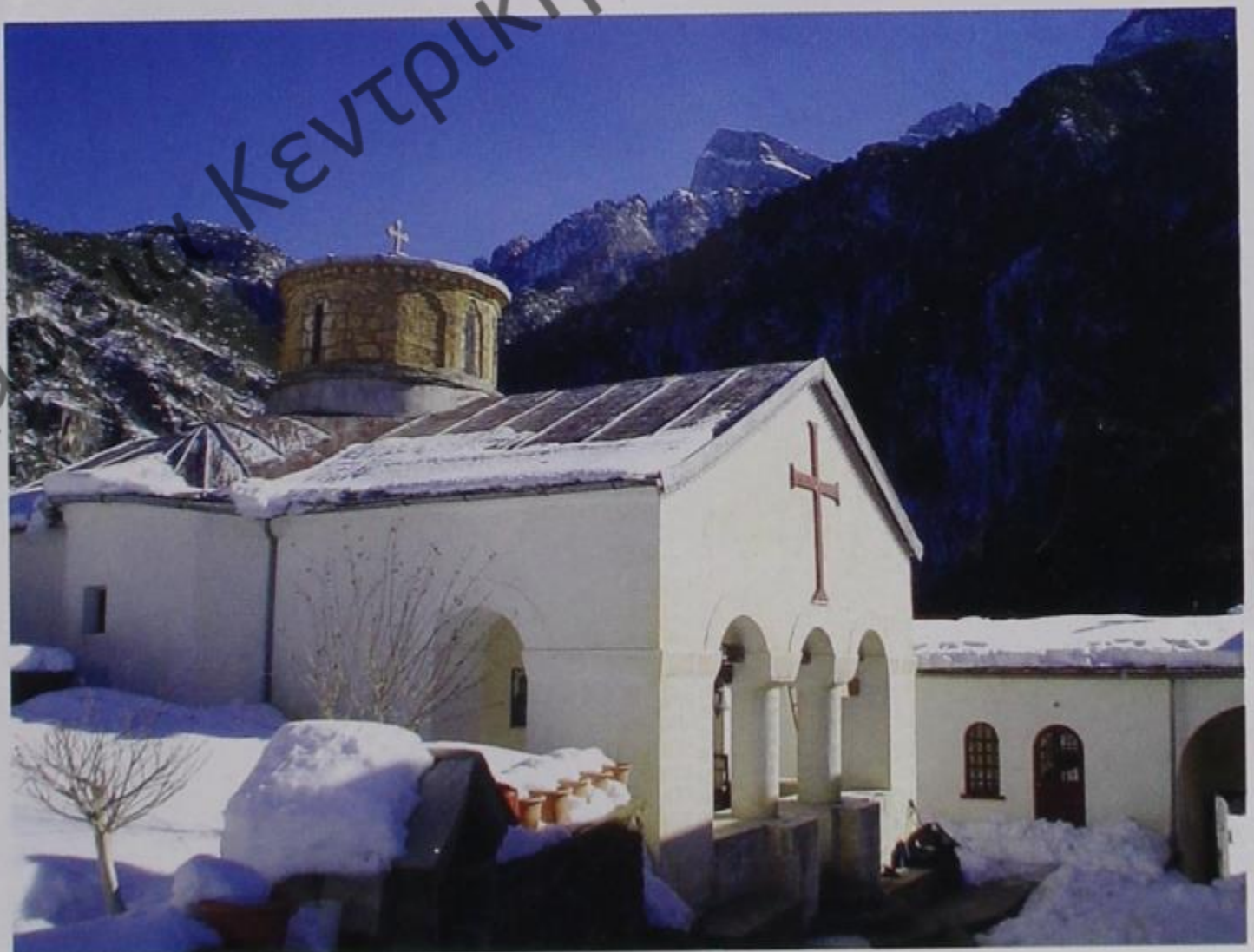
The nave of Panagia Stomiou monastery in the Aaos gorge
