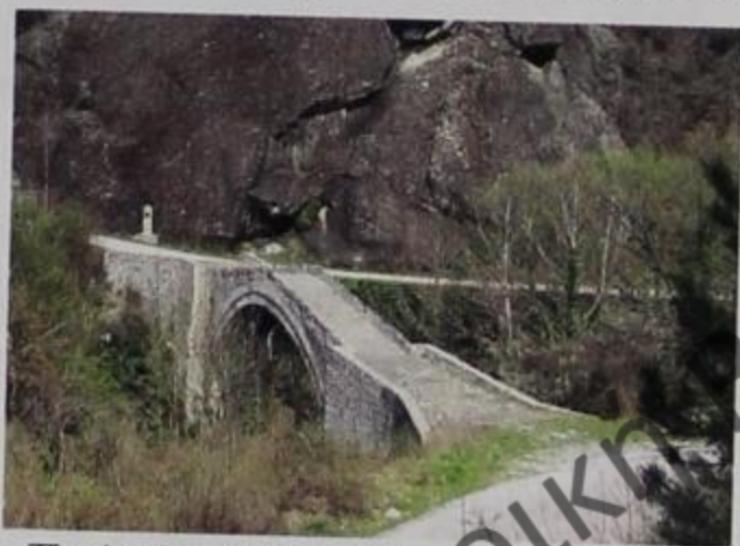
The bridge of Mavri Petra close to Pournia
