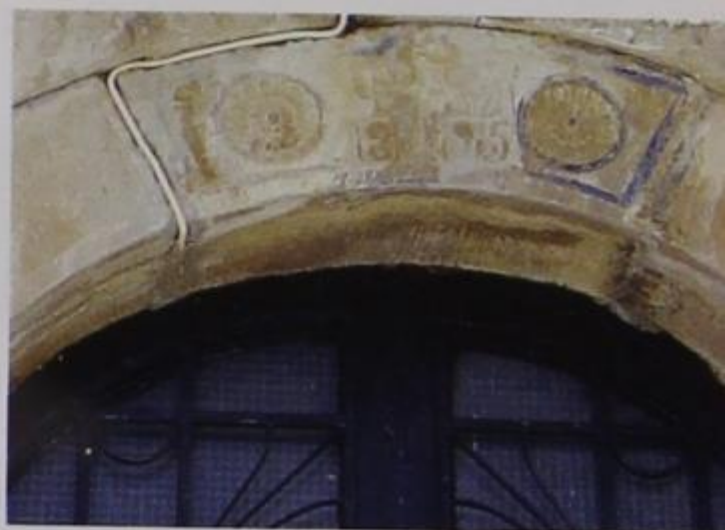
An engraved key stone of a house entrance
