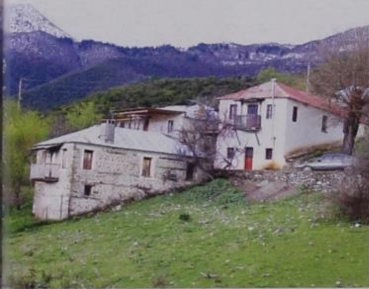
Typical houses in Pyxaria
