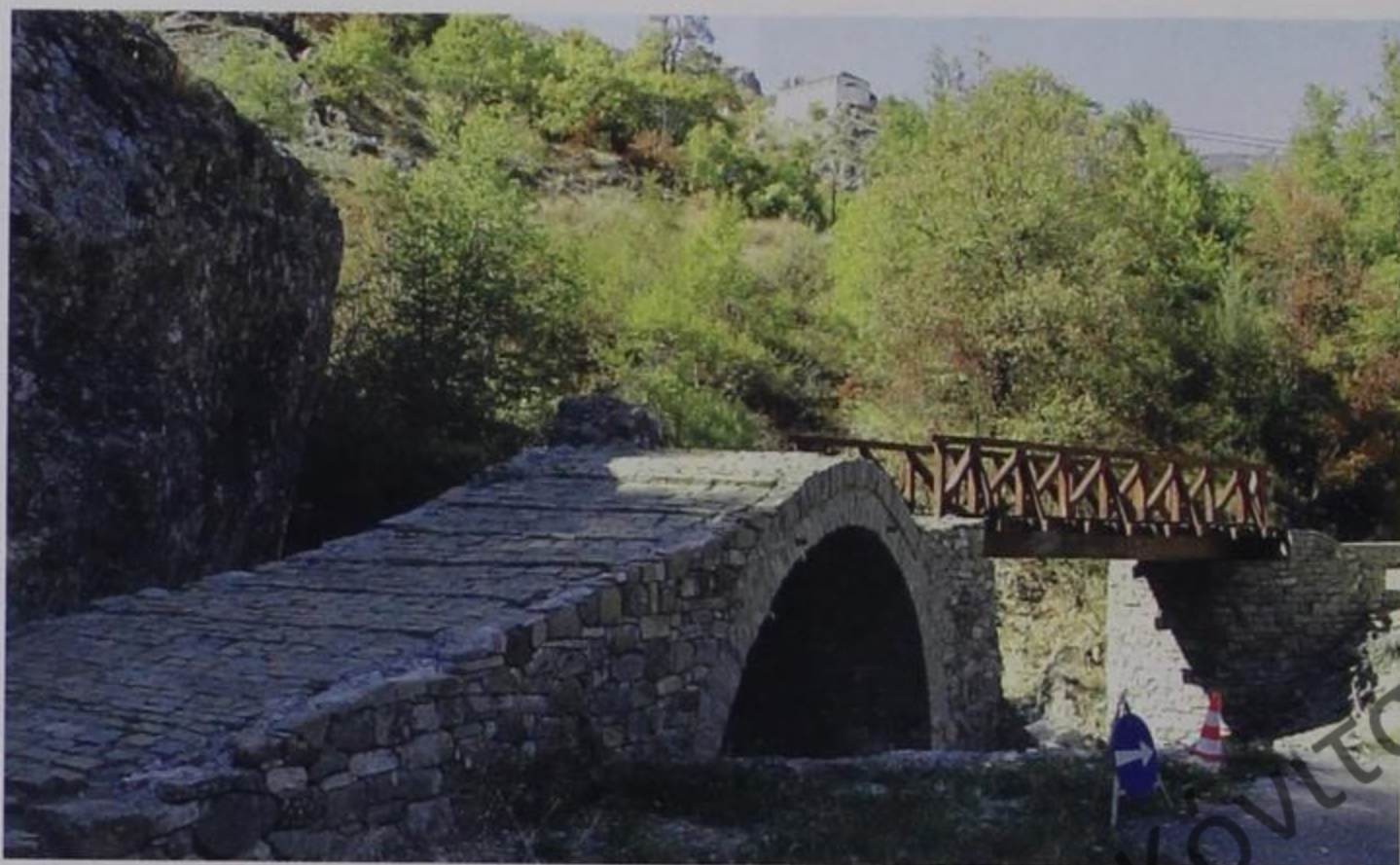
The small bridge at Paraspori location, Hioniades
