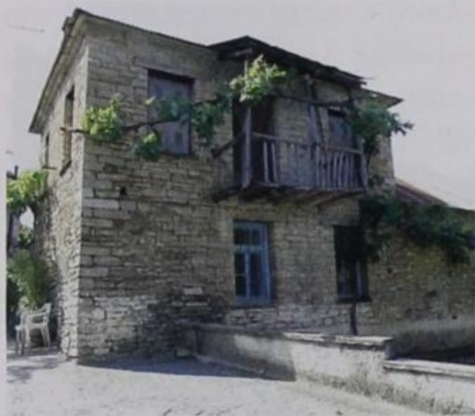
A typical house in Exohi
