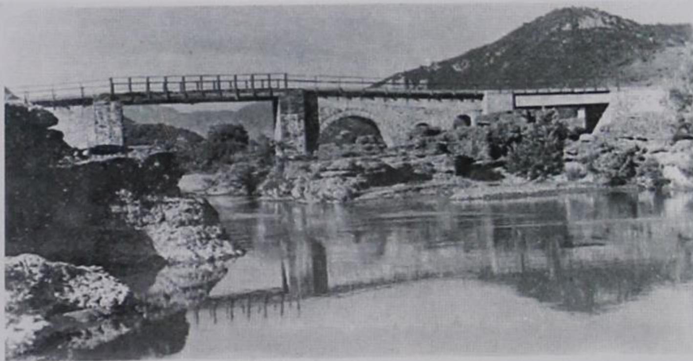
Mesogefyra bridge during the WW II.
