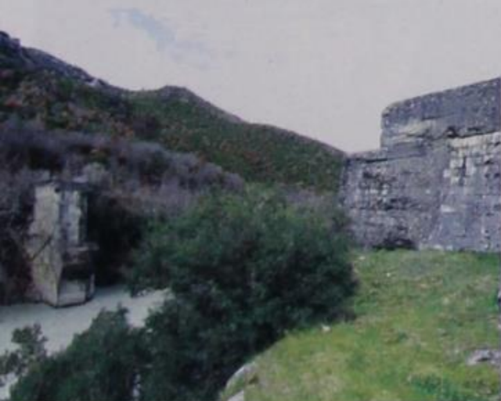
The pedestals of Merziani bridge today
